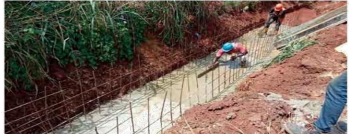
DRAINAGE BASE CONSTRUCTION
