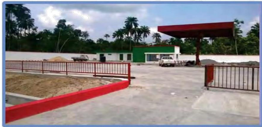
CNG Station for NIPCO PLC at Amuokolo Delta State
