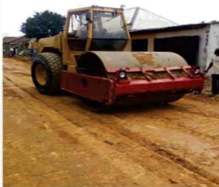
Construction of Itam Market Road
