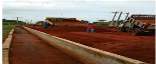
EARTHWORKS IN PROGRESS
