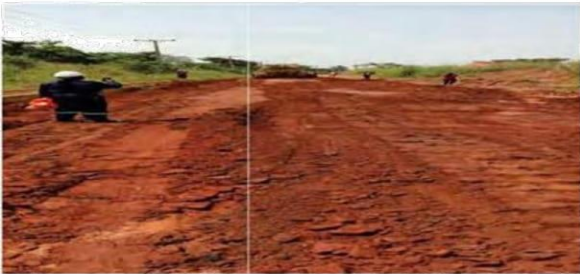
CLEARING OF SITE IN PROGRESS
