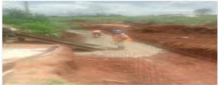
CONCRETE BASE CONSTRUCTION
