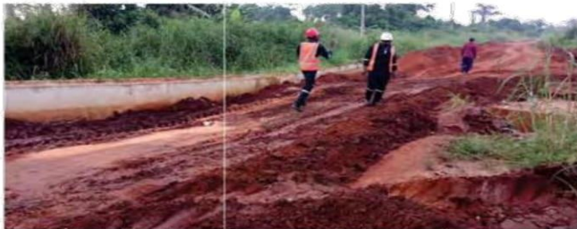
EARTHWORK IN PROGRESS
