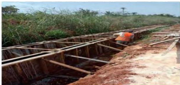
INSTALLATION OF FORMWORK
